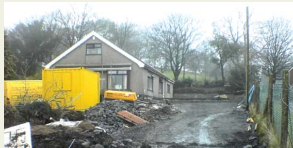
Original Property & Site
