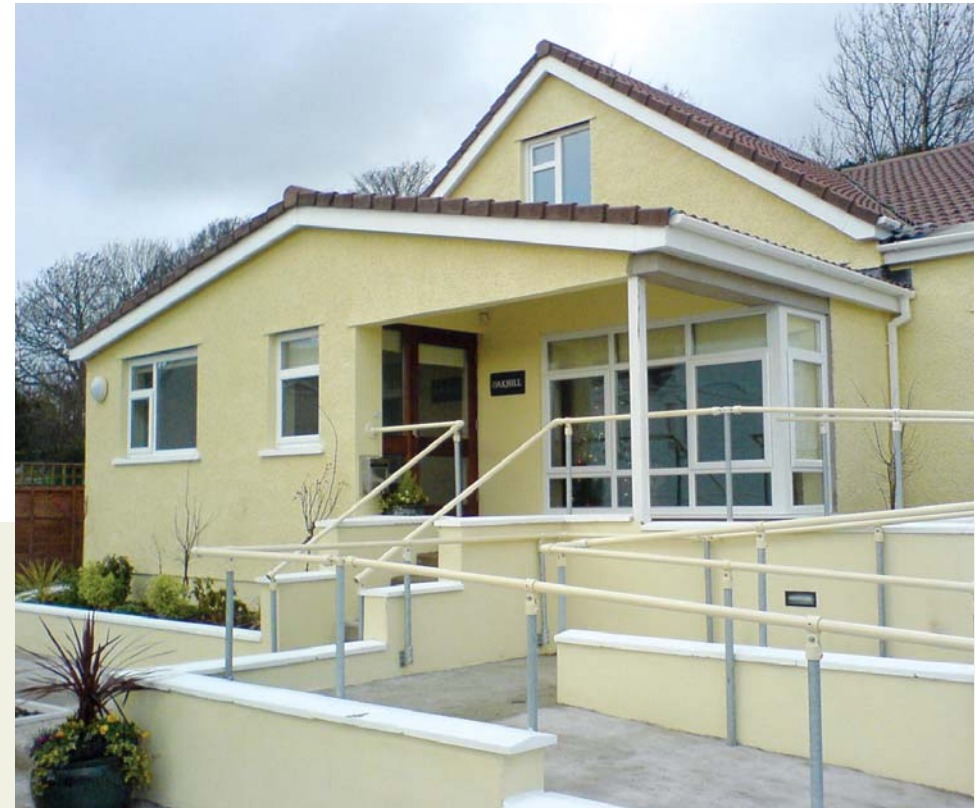
The Front Facade
